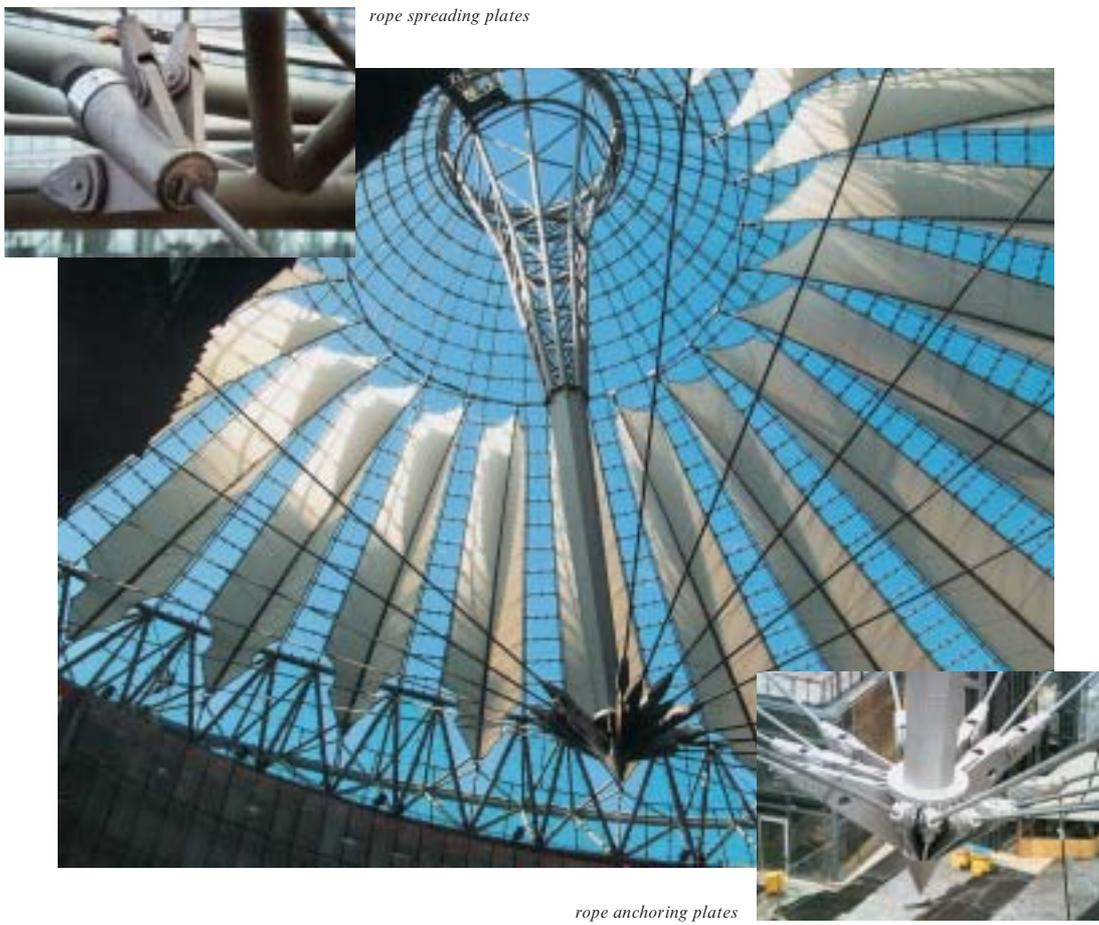
**Figure 15:** Roof structure of the Sony-Center in Berlin, with DILLIMAX 690 straps for carrying beams, rope spreading and rope anchoring plates
